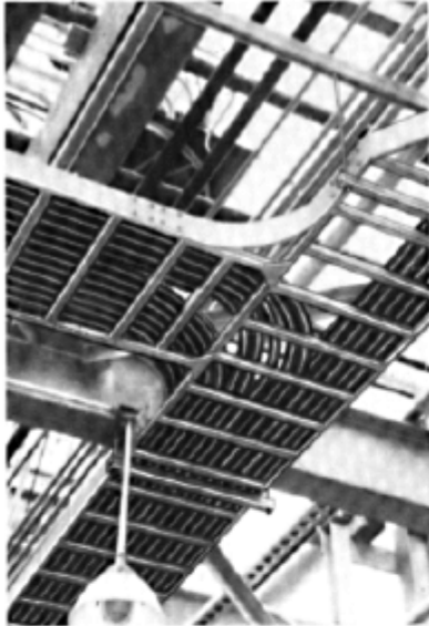
Figure XI Typical tray arrangements are similar to instrument tubing or electrical cable tray.
