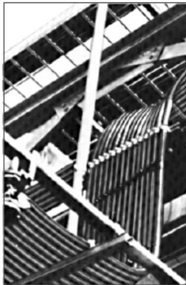
Figure IX Multiple groupings require 1/2” or more spacing to allow for heat dissipation.
